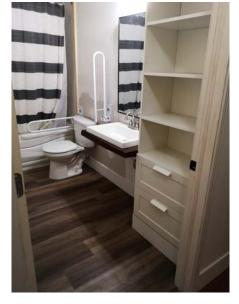
to install a 36" door, a bathroom linen closet was replaced by the 13" deep shelving/drawer unit, grab bars were installed to allow transfer from wheelchair to toilet, and the original basin and larger vanity were replaced by the one shown which permits wheelchair access. New flooring was installed.
